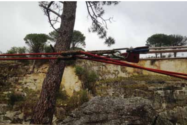
High line tensioning system
